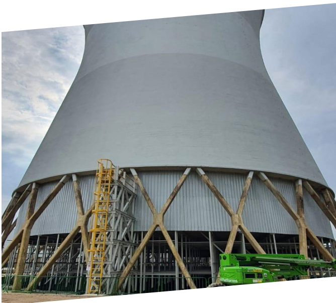
Natural Draft Cooling Tower revamping activities in UK
