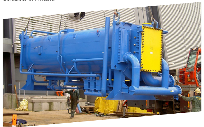
Absorption Chiller in Sweden
